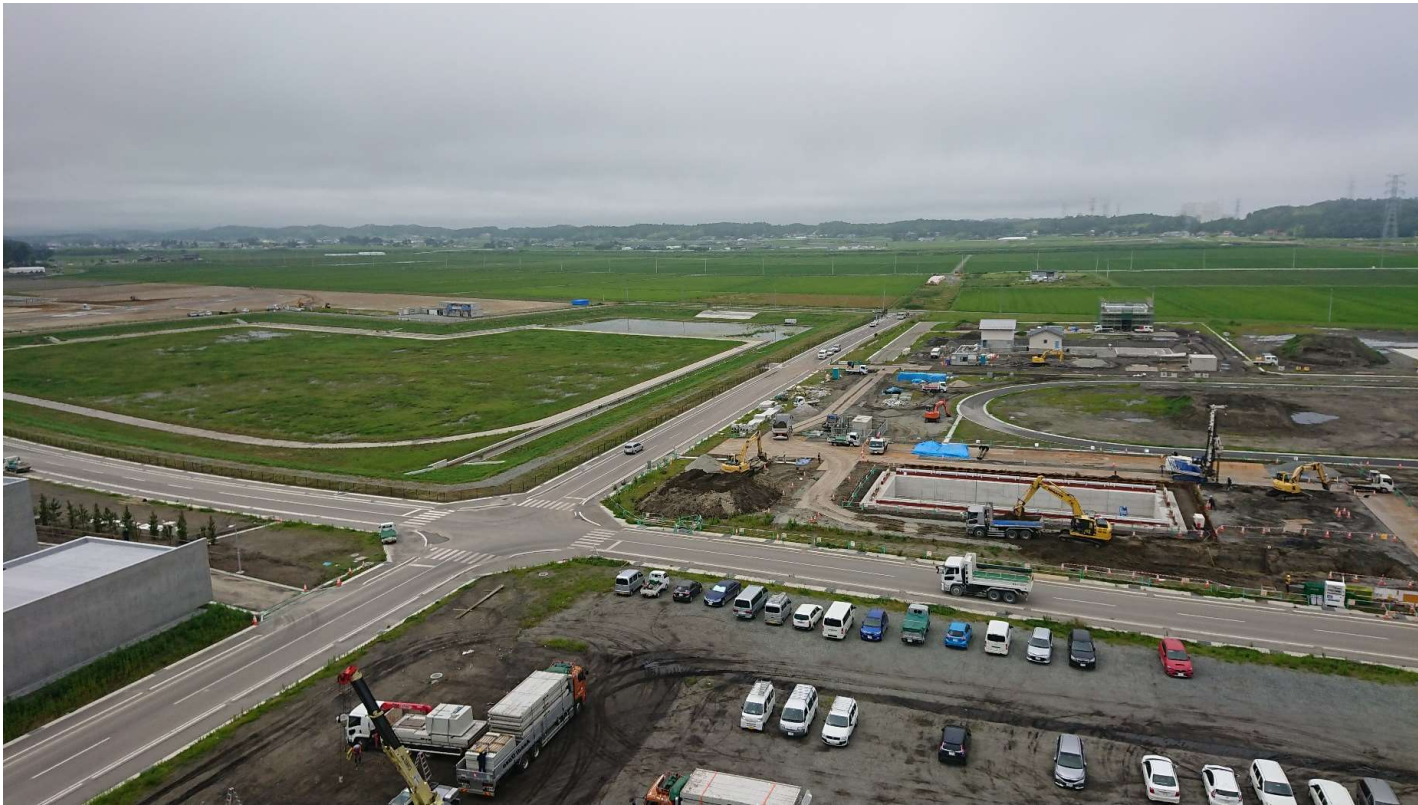
Debris/landslide test field
